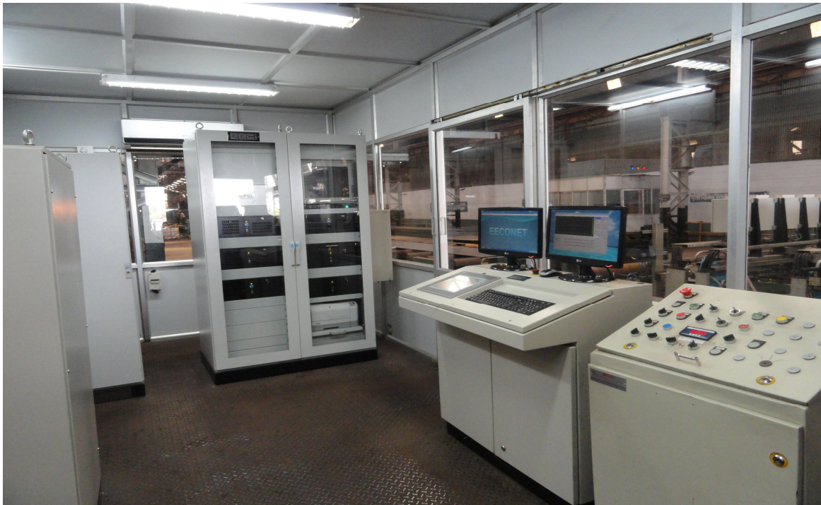
The above photograph shows Electrical Panel having PLC unit, Electronic Panel containing industrial PC, HMI Control & Mechanical Control Panel. All these are installed in the Operator Cabin.
