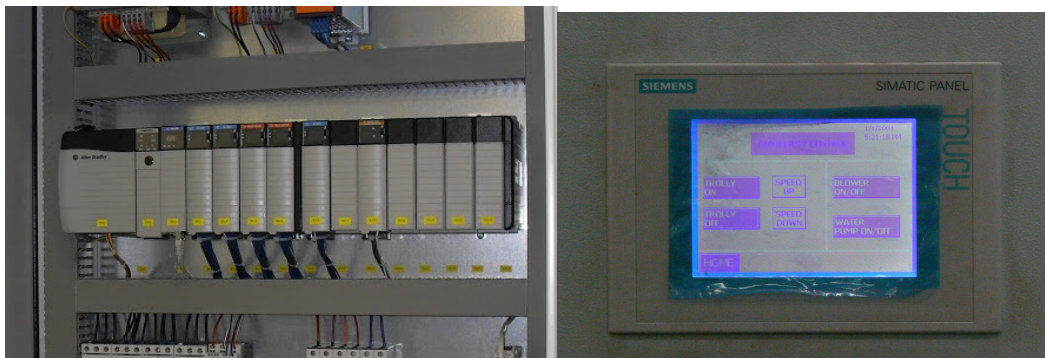
PLC & HMI control system
