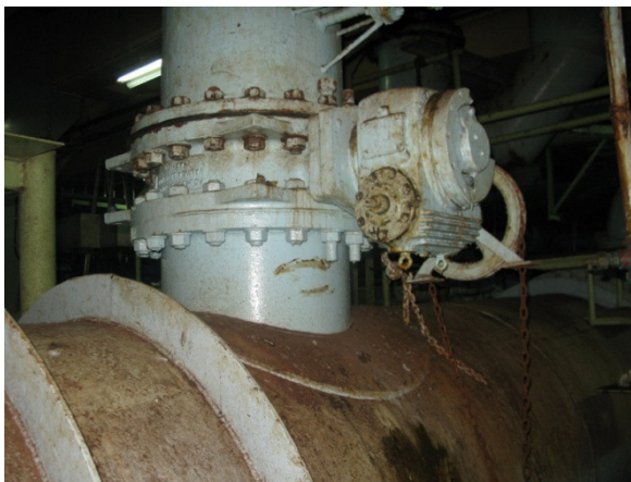
Fig.1-Chain & wheel operated butterfly valve the heat exchanger (PW/SW Hx #5)
