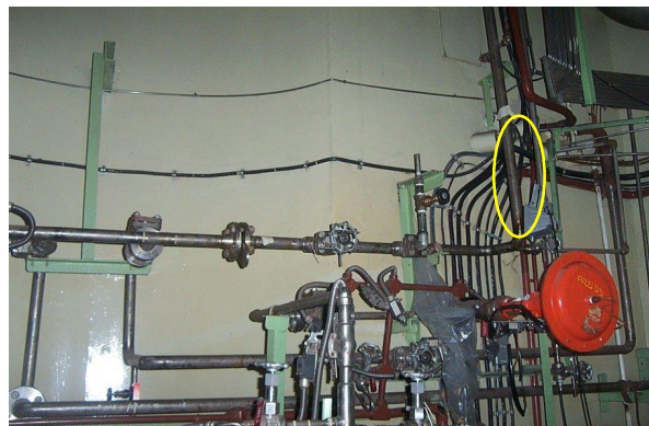
Fig.7 Choked line marked
