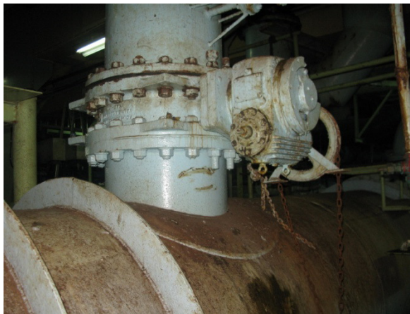
Fig.1-Chain & wheel operated butterfly valve
