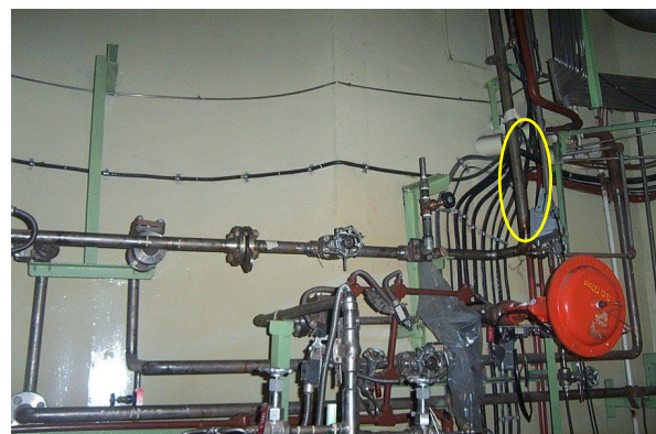
Fig. 7 Choked line in the extent of the line.
